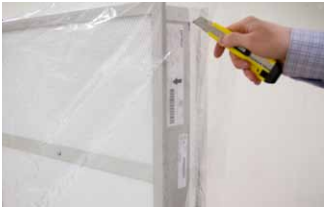
C) Cut plastic bag and remove with care. Do not cut along the filter face or insulation.
